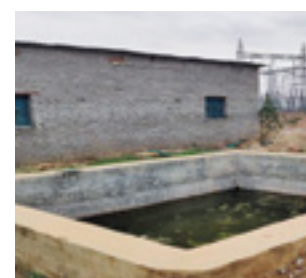
Construction of Surface Water Storage tank with concrete cubes, Madhya Pradesh
