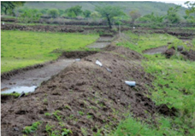
Farm Bund (FB) with pipe outlet
