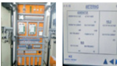
AVR PANEL WITH DIGITAL EXCITATION CONTROL
