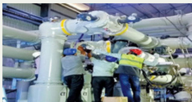
Photos during Restoration
