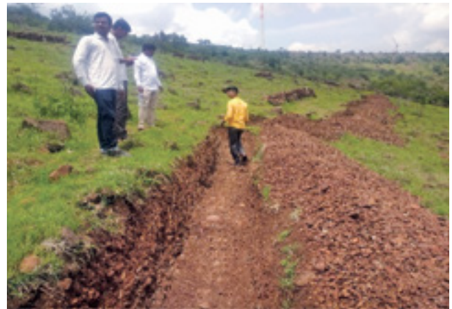
Water Absorption Trench (WAT)
