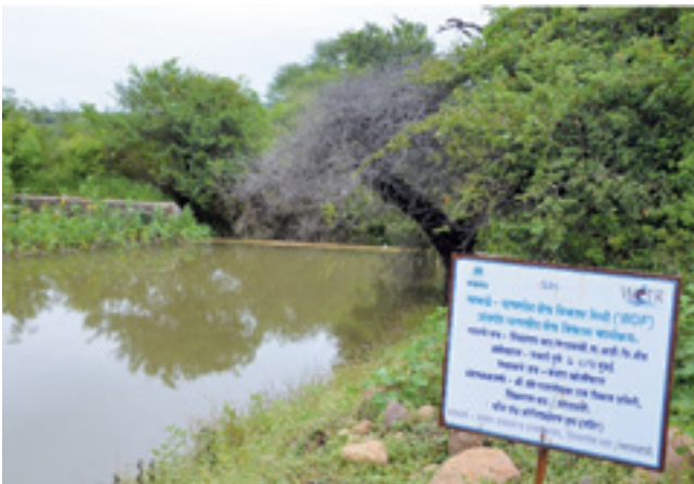
Water stored in de-silted Check Dam
